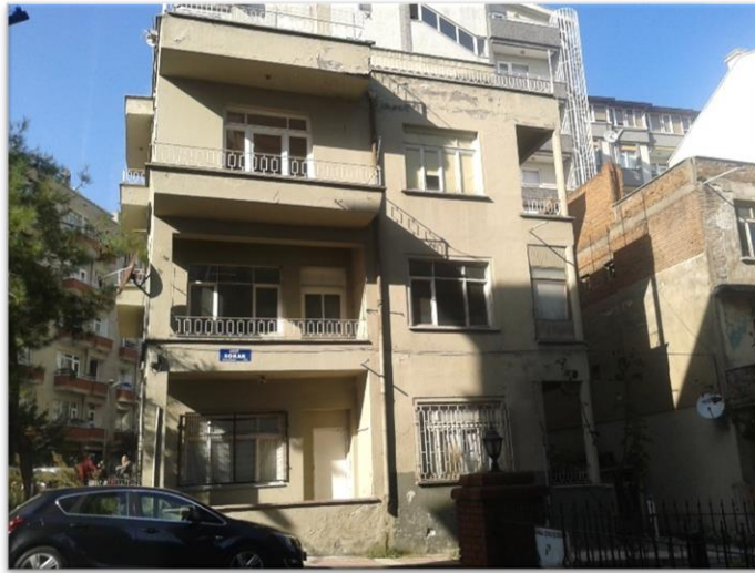
Fig.6. Abandoned lodging buildings
