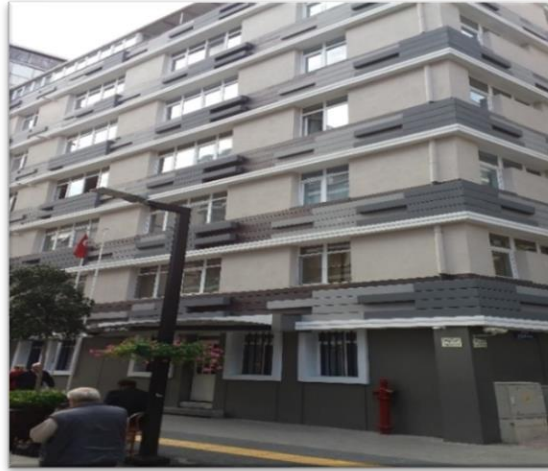
Fig.1. A law enforcement building featuring exterior thermal insulation cladding
