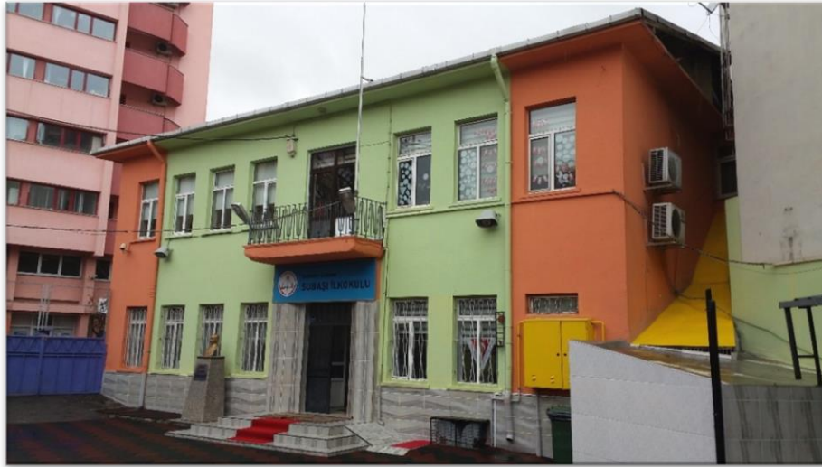
Fig.5. A school building with regularly maintained exterior facades
