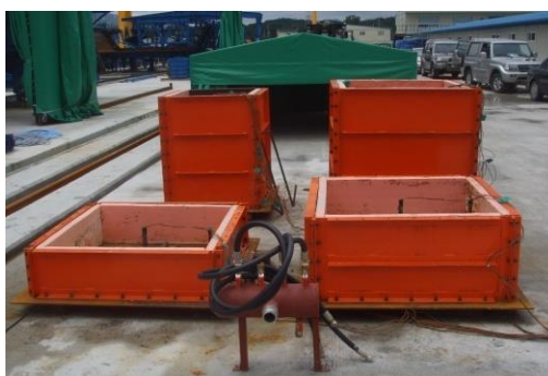
Photo 1. Formwork for mock-up test
