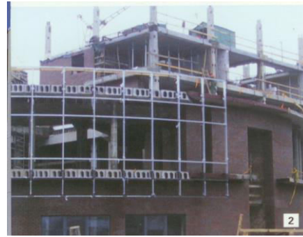
2. Residential building with commercial Premises, during construction, in Klaipeda, Lithuania
