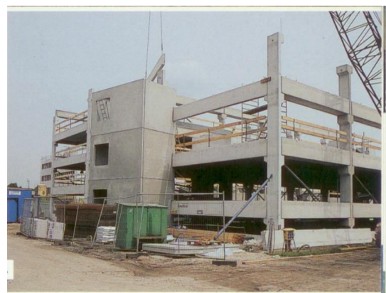
4- Car park in Leusden, The Netherlands
