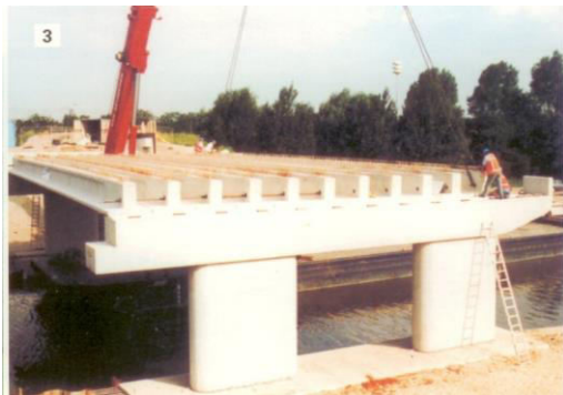
1. Road bridge in Alphen a/d Rijn, the Netherlands
