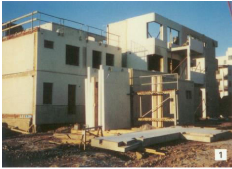
1. Precast structure for a residential building: walls, core, floors and stairs
