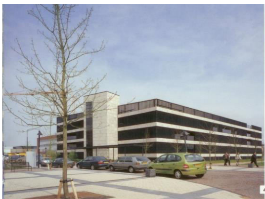
3- Car park at Ericsson in Gothenburg, Sweden
