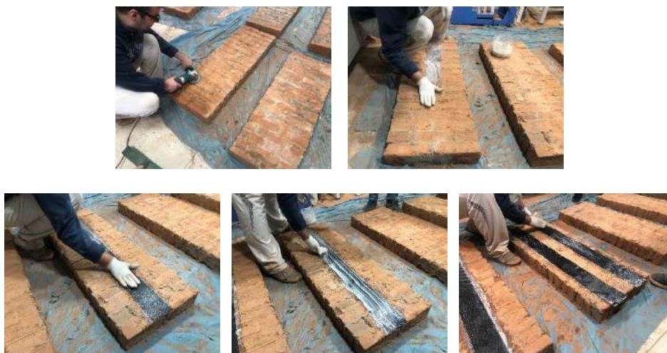
Figure 5. Strengthening processes of masonry panels [30]
