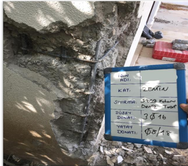
Fig.4. Concrete chipping process in columns
