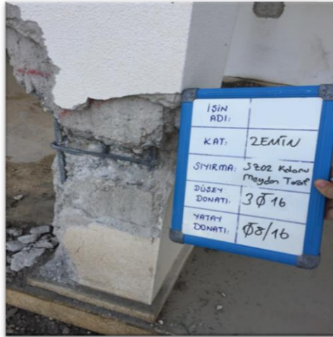
Fig.5. Concrete chipping process in columns
