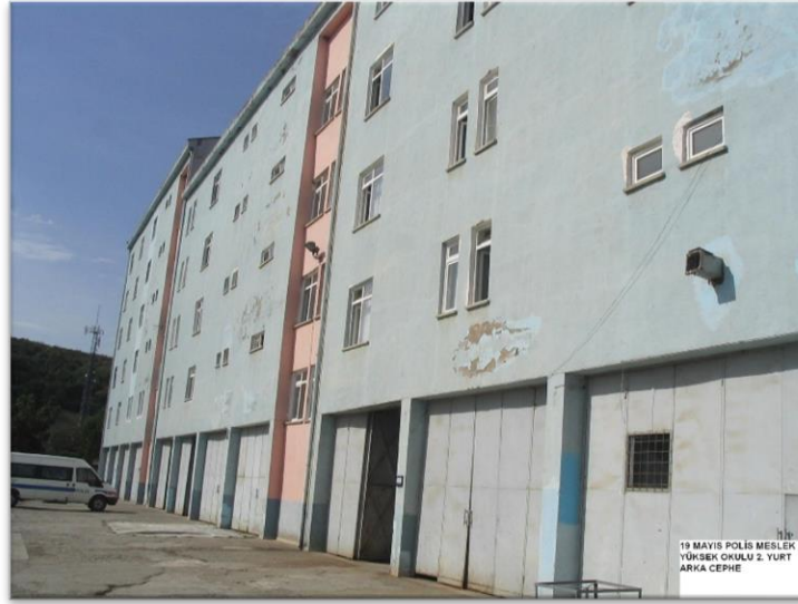
Fig.8. A public building with a ground floor utilized as a garage
