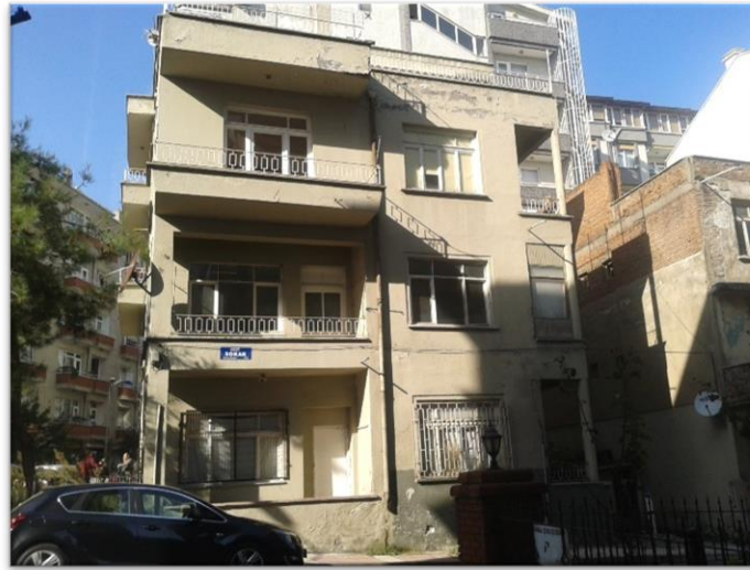
Fig.6. Abandoned lodging buildings
