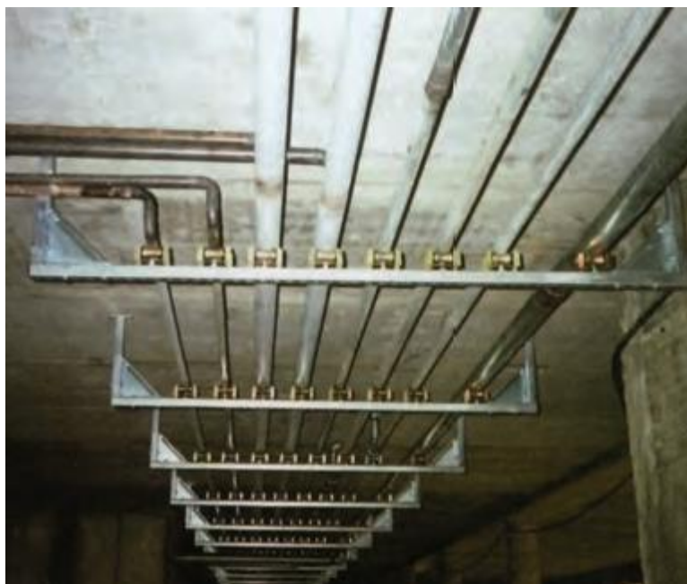
Fig. 3. Fastening of channels on compensation rollers [11]
