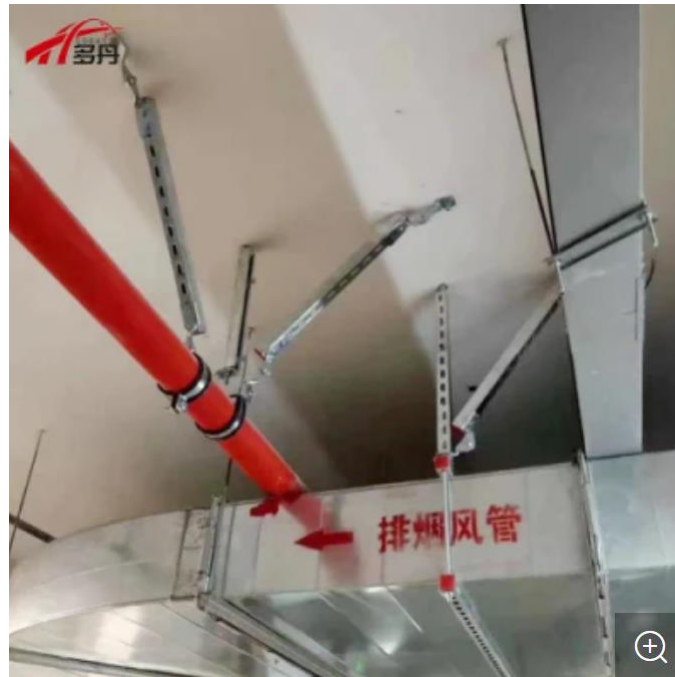
Figure 1. Suspension Seismic Bracing System Steel Support for HVAC Duct [9]
