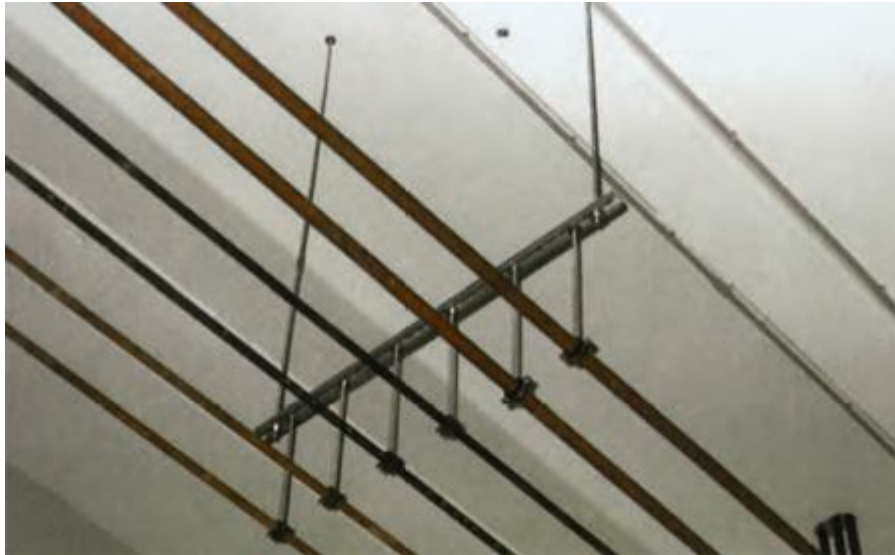
Figure 4. Seismic suspension of pipelines [11]
