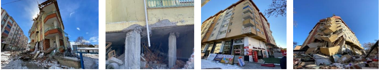
Figure 12. Examples of damages in structures with torsional irregularity [10]
