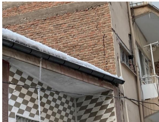
Figure 13. Two masonry buildings with adjacent layout and not the same number of floors (38,35371 N, 38,32353 E) [17]
