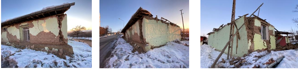
Figure 17. A masonry structure that combines the causes of the corner collapse mechanism (38.31279 N, 38.25054 E) [17]
