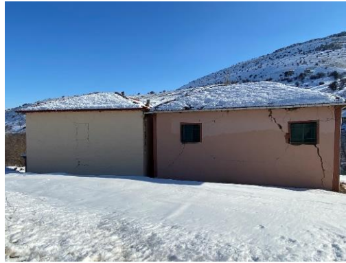
Figure 12. A 2-storey masonry building (38,38479 N, 37,95899 E) [17]
