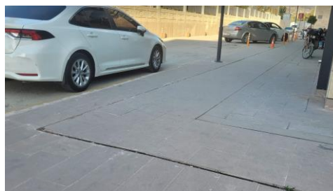
Figure 8. The hinged platform covers of the seismic gaps along the perimeter [11]
