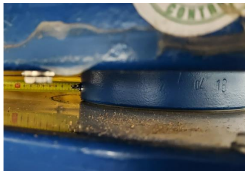
Figure 7. Measured isolator bottom plate displacement at Hatay Dörtyol Hospital [11]
