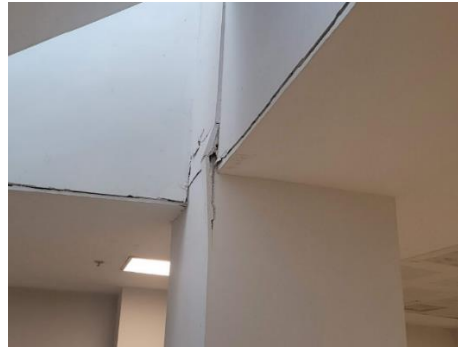
Figure 1. Cracking and slight damage in gypsum boards covering the seismic isolators due to displacement during the earthquakes [10]
