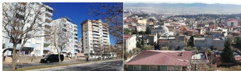
Figure 16. Buildings on the hillside of Kahramanmaras city center; a) (left) new high-rise RC frame buildings with no/slight damage, b) (right) old and low-rise RC and masonry buildings that performed relatively well during the earthquakes (courtesy of the EEAT) [19]
