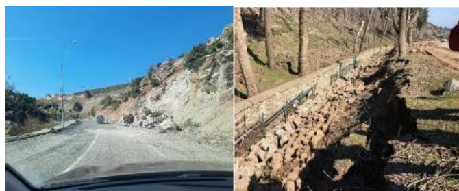
Figure 8. a) Rockfall on the road route around Nurdagi, b) damages due to lateral spreading along the stream channel in the Fevzipasa neighborhood of Islahiye [19]
