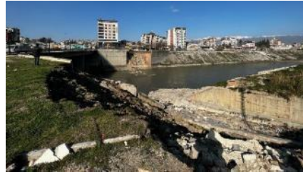
Figure 9. Settlements in alluvial soils along the Asi River in Hatay and damage to retaining walls due to lateral spreading [19]
