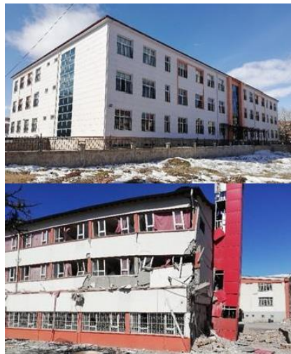
Figure 18. a) A school building with no damage in Golbasi (Adiyaman), (top) b) a severely damaged school building in Kahramanmaras city center (bottom) (courtesy of the EEAT) [19]
