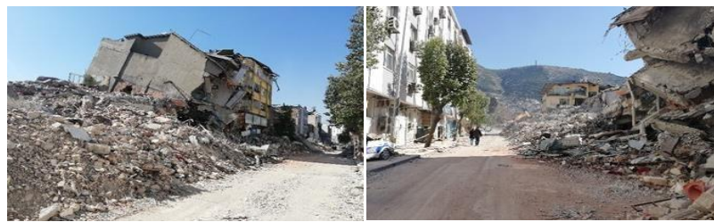
Figure 12. The photos of total destruction in Antakya, Hatay (courtesy of the EEAT) Antakya city was recognized for its cultural diversity and richness and it resided many historical structures, including invaluable heritage belonging to different religions. Unfortunately, most of these structures were either severely damaged or collapsed during the sequential earthquakes of February 2023 in Turkiye (Fig.13) [19]
