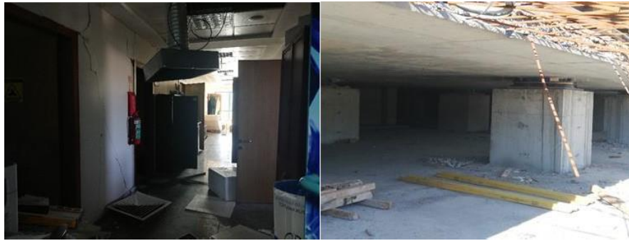
Figure 17. a) Existing city hospital in Kahramanmaras with extensive non-structural damage, b) a new hospital construction in Kahramanmaras with base isolation system (the isolators worked and performed well during the earthquake although most of them were not installed yet) (courtesy of the EEAT) [19]
