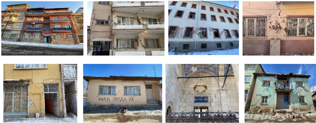
Figure 13. In-plane damages in masonry structures in Malatya [10]
