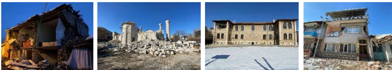
Figure 13. In-plane damages in masonry structures in Malatya [10]
