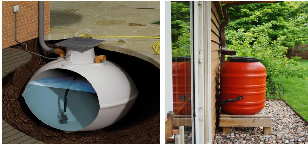
Figure 2. Underground tank systems collect roof runoff for watering plants Source: Meg Calkins, the sustainable sites, 2012 [6]
