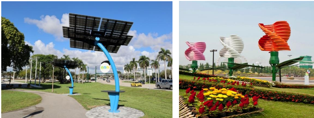
Figure 1. Energy efficiency and reduction of power transmission costs for sustainable parks through solar panels and vertical axis turbines Source: Meg Calkins, the sustainable sites, 2012 [5]
