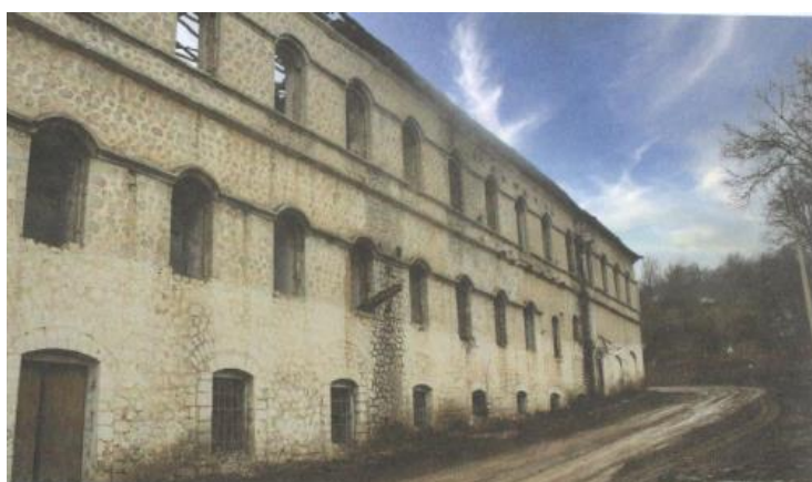
Figure 34. The Building of Shusha Hospital, after the occupation (Shusha the Cultural Capital of Azerbaijan, 2022)
