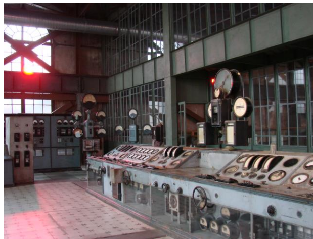
Figure 17. Central İstanbul – Views from the interior
