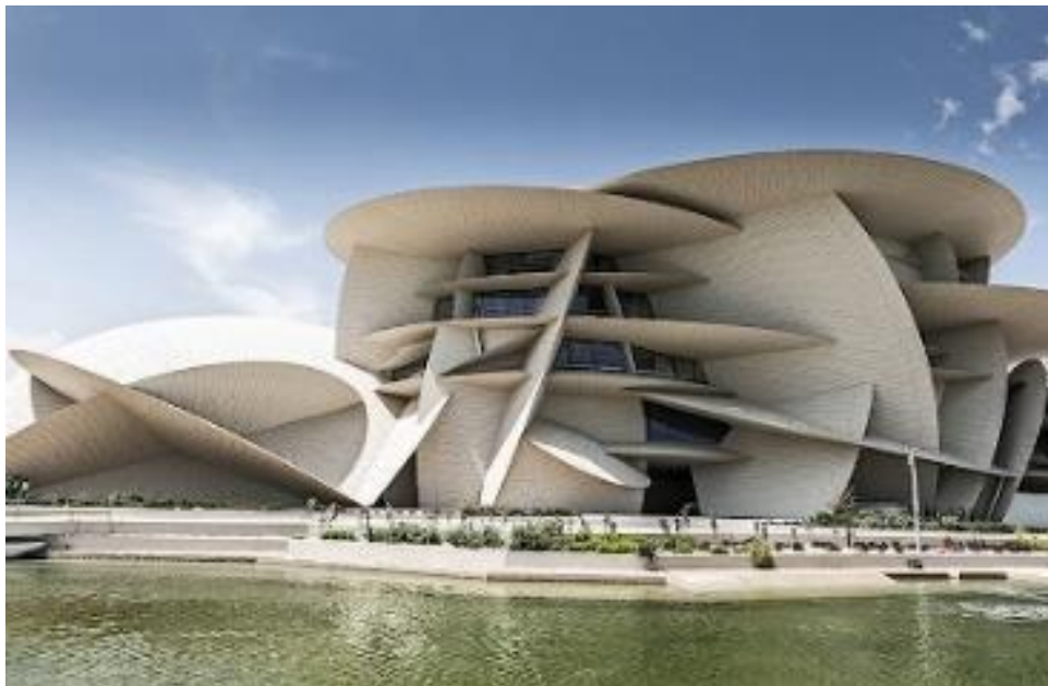
Figure 4. National Museum of Qatar. Architect Jean Nouvel ( https://architime.ru/news/nuvel/national_museum_qatar.htm#1.jpg )
