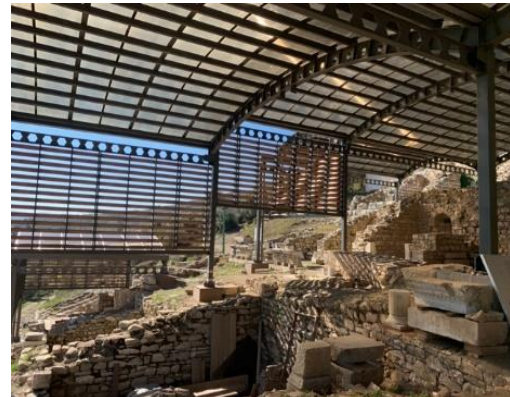
Figure 17, 18. The Protection Roof placed on the Roman Bath Ruins in Metropolis (Tanac Zeren Archive)
