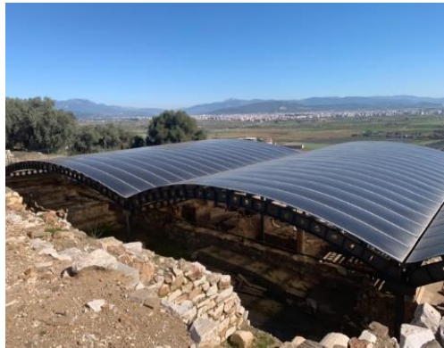
Figure 17, 18. The Protection Roof placed on the Roman Bath Ruins in Metropolis (Tanac Zeren Archive)
