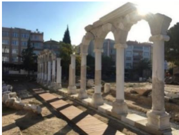
Figure 5. The Anastylosis Work of Columns (Tanac Zeren Archive)
