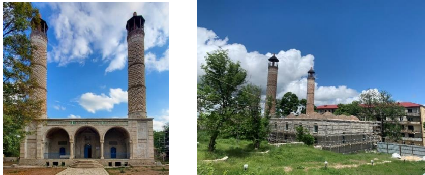
Figure 6 c, d. The upper mosque of Gevhar Agha after so called ‘restoration’ in the last years of occupation and today [picture by author]
