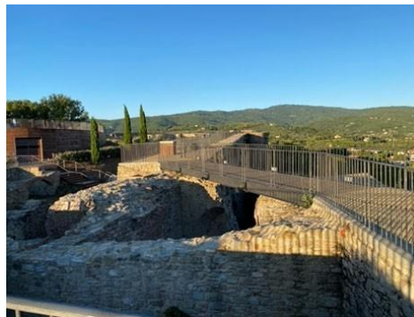
Figure 27. A new bridge over the “Belvedere Bastion” destroyed in 1800 by the Napoleon troops
