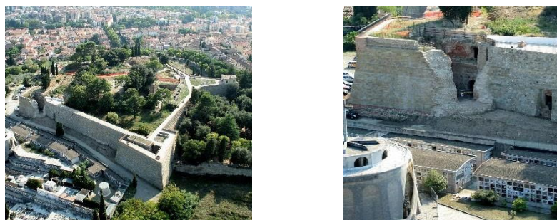
Figure 19, 20. The Fortress after the restoration of the external walls, aerial views (end of phase one)
